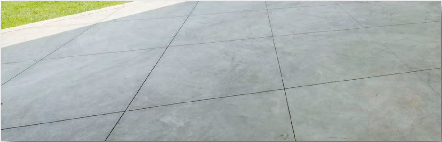
PORCH FLOOR: SMOOTH FINISH CONCRETE WITH EQUALLY-SPACED CONTROL JOINTS, DIAGONAL SAW CUT IN PATTERN
