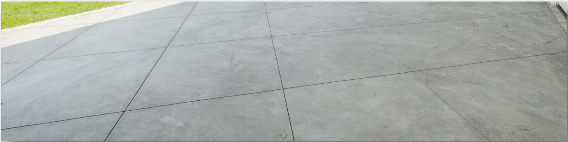
FRONT PORCH FLOOR: SMOOTH FINISH CONCRETE WITH EQUALLY-SPACED CONTROL JOINTS, DIAGONAL SAW CUT IN PATTERN
